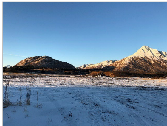
Exhibit 1-1: ADQ runway and taxiway, facing south.
